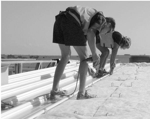
Figure 2.5.F Clips Located Over HiKlip® 630 Male Rib
